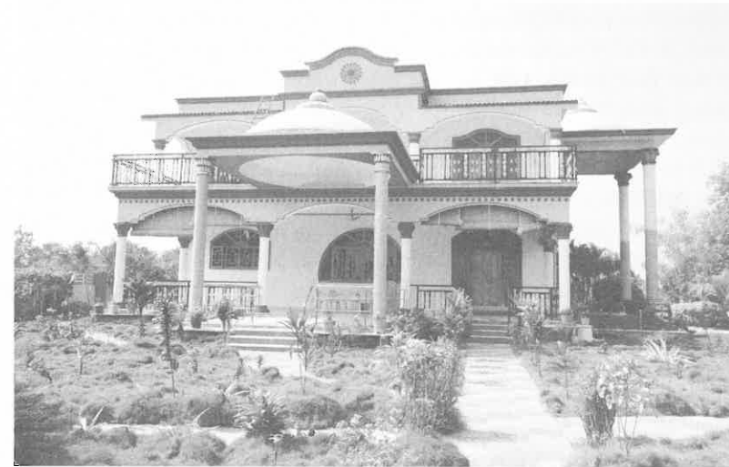
Photo 8 Rao's village mansion, Bhadrachalam Photo by Dale Benbabaali.
